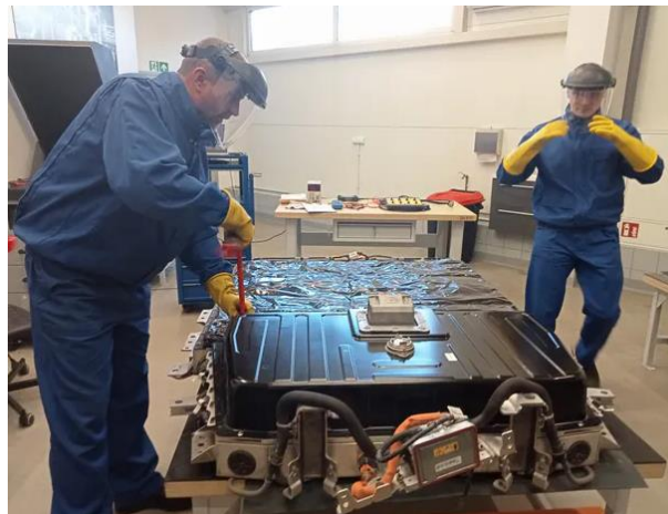
Authorized Repair Plant of Traction Batteries for Renault Electric and Hybrid Cars in Zabrze.
